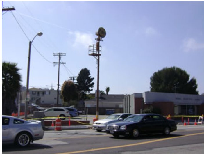
This civil defense siren was discovered by Caltrans engineers on State Route 1 (Lincoln Boulevard) in the Westchester area of Los Angeles.
